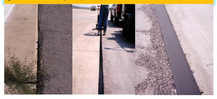
Sealant won't take the bump out of a bridge approach. Hot Mix Skin patch wont last. Mastic repairs work great.
