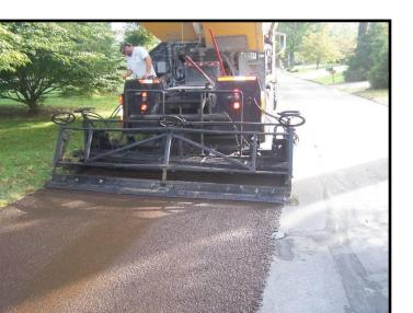
In Preparation for a Micro, Slurry or Thin Overlay you must treat the cracks or they will reflect through quickly.
