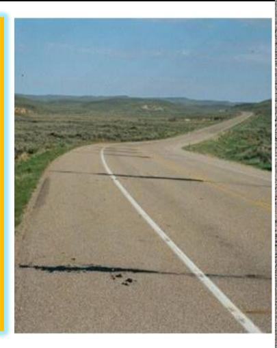
Mastic will seal and bridge the depressions that are wider than the crack.
